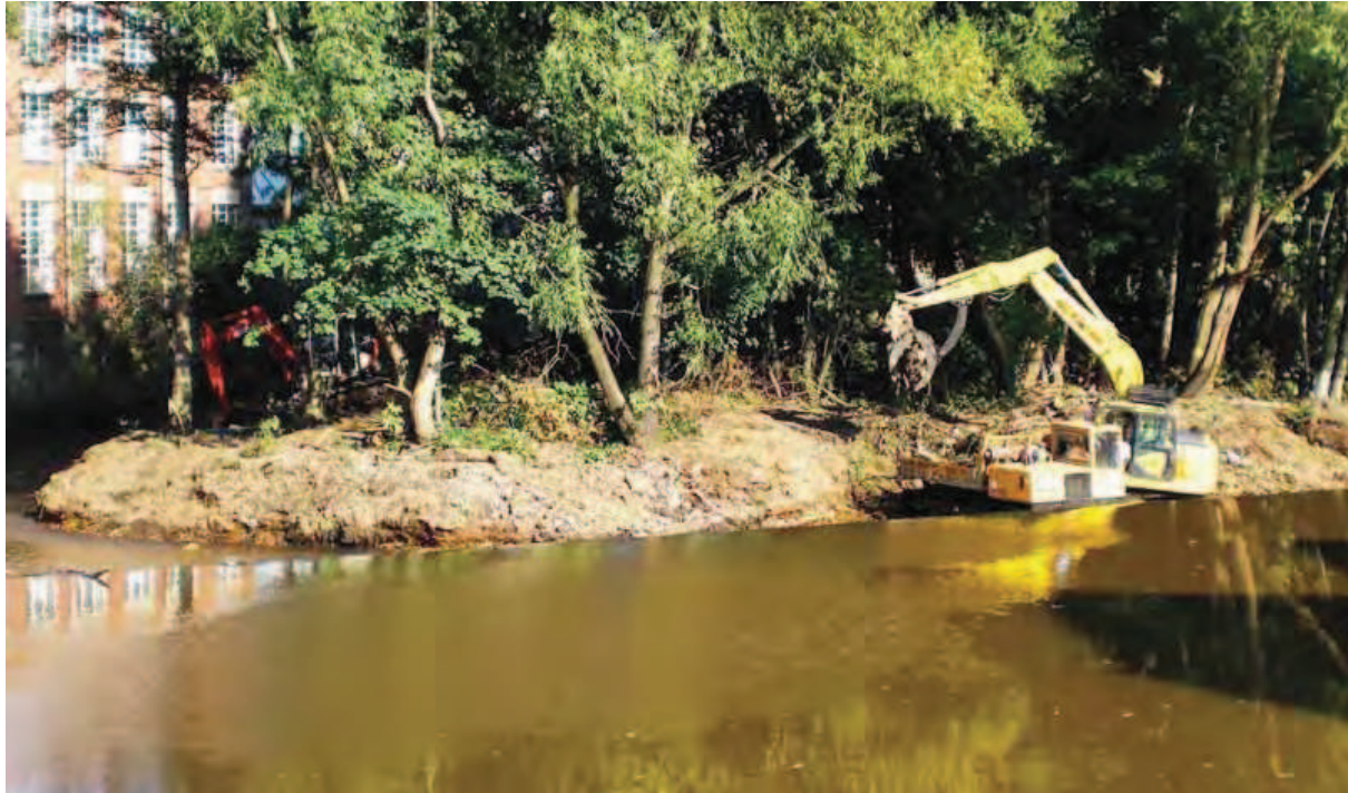
Work by the Environment Agency at Kelham to reduce flood risk by clearing the river channel obstructions. Habitat improvements were made at the same time
