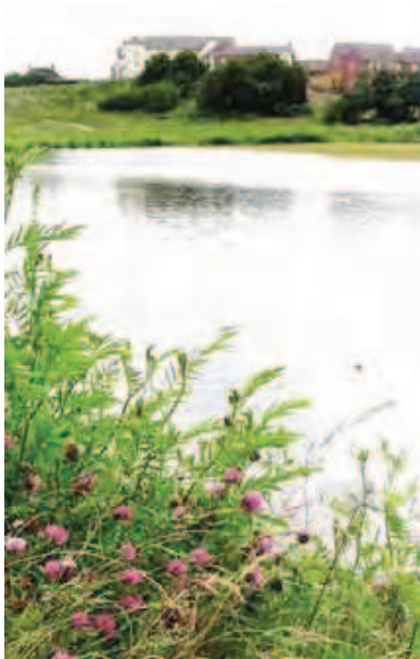
Sustainable drainage. A flood storage basin at the manor holding water after the rainstorm that caused Sheffield's floods in June 2007 Photo Credit: Roger Nowell
