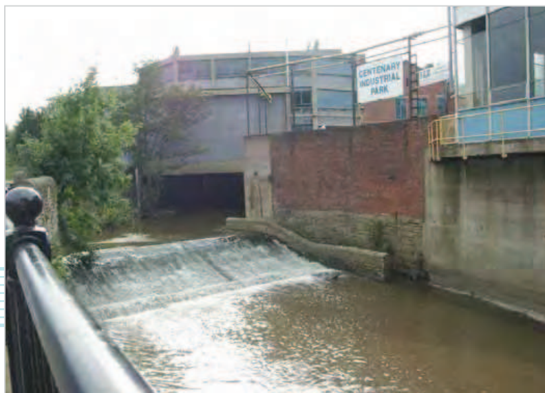
In many places, the rivers have been heavily engineered, this is the Sheaf on Little London Road
