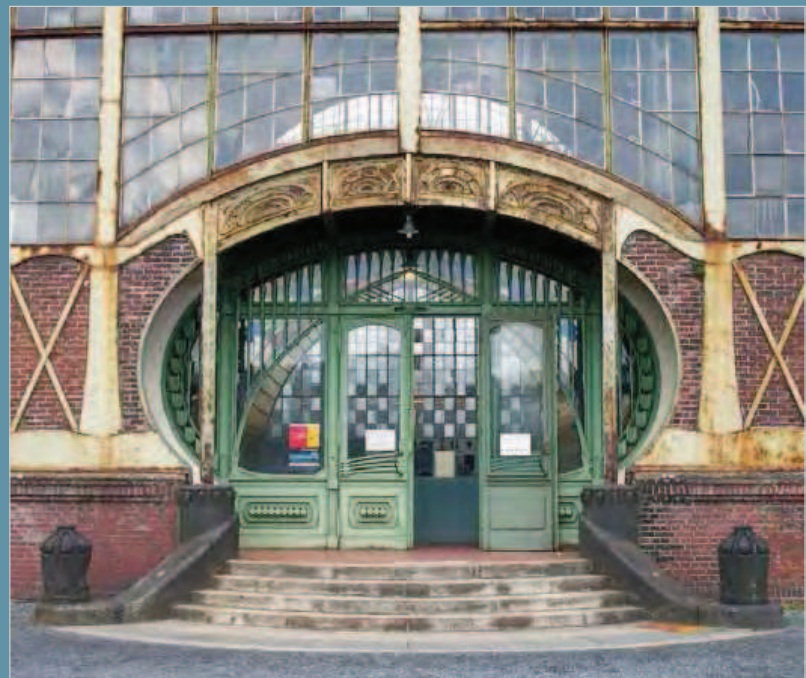
Re-used structures that could easily have been cleared away as derelict Photo Credit: Tom Wild
